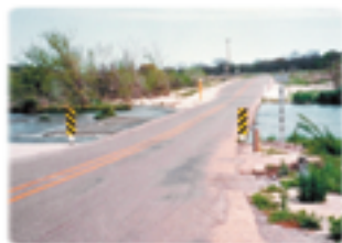
IRS Hazard Markers are perfect for low water crossings.
